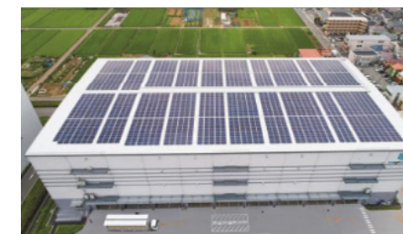
A solar power generation system in a logistics facility owned by the company
