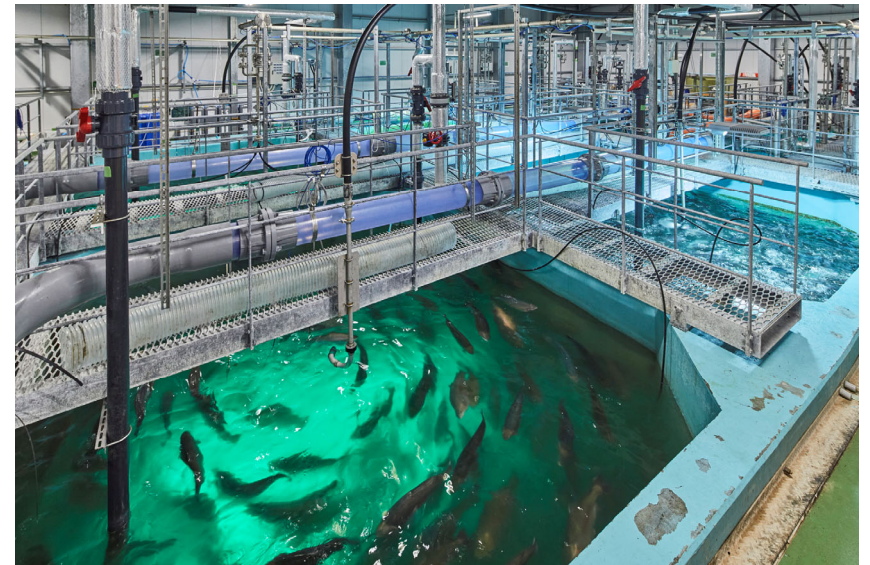
▲ Closed recirculating land-based aquaculture system in operation
