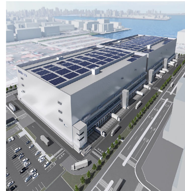
▲Artist's rendering of cold storage warehouse after rebuilding (scheduled for completion in FY2027)
