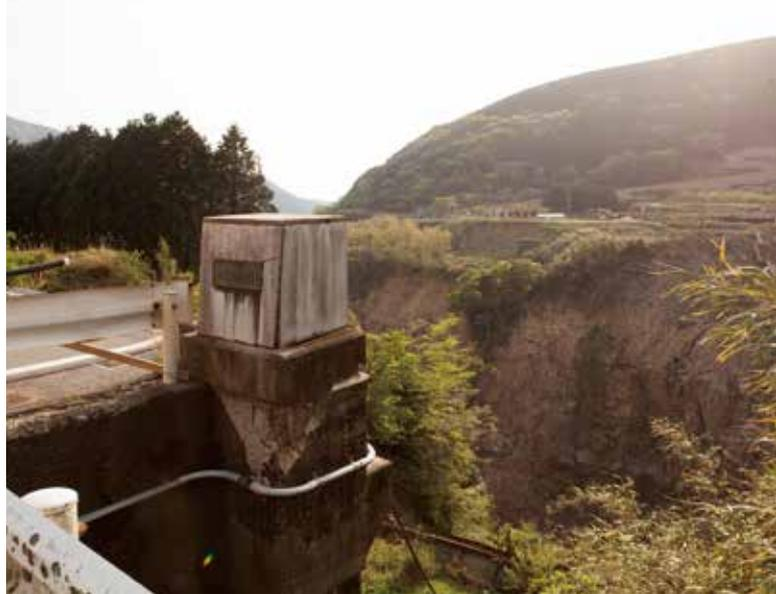
Tateno district cut off by collapse of Aso Ohashi Bridge due to landslides
