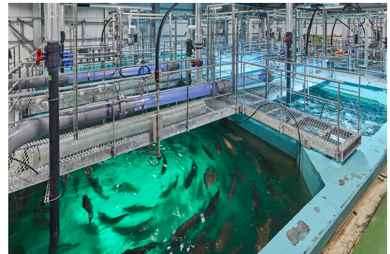
▲ Closed recirculating land-based aquaculture system in operation
