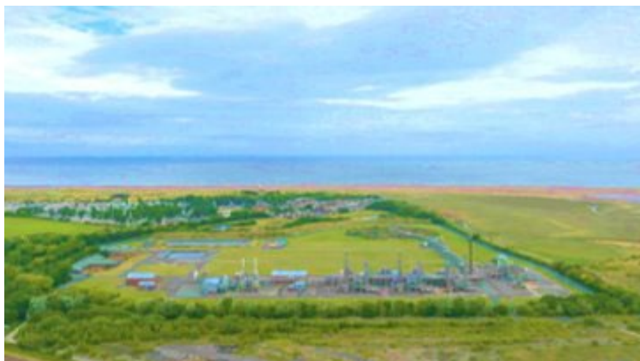
CO 2 transportation and storage facilities related to the project
