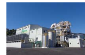
Power generation plant
