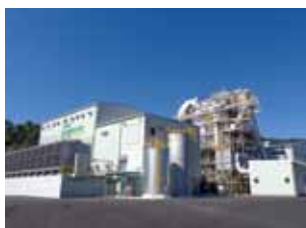
Electric power station of a Fund recipient
