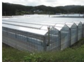
Steel pipe greenhouses funded by the reconstruction fund
