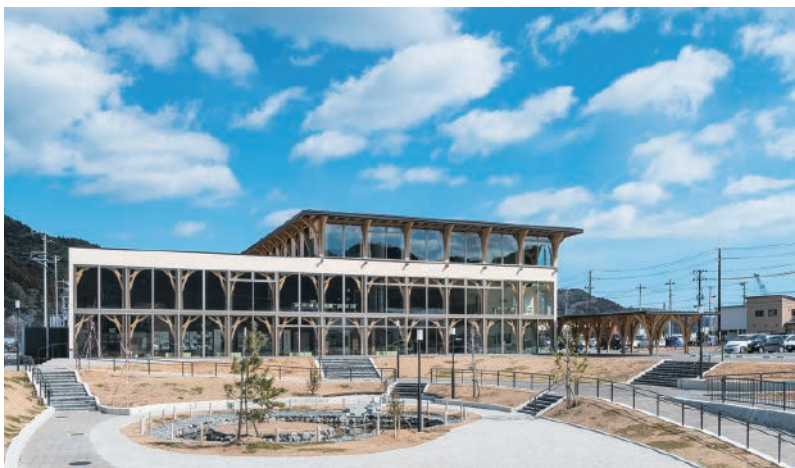
The Bunka-Karyu (cultural interaction) Center of Otsuchi Town in Iwate Prefecture is a large-scale three-story glass-walled wooden building
