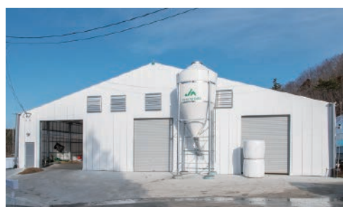
The cattle facility was built as a property of litate village.
