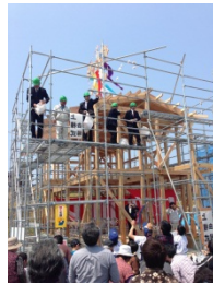
Ceremony for the completion of frameworks of public wooden houses for disaster sufferers
