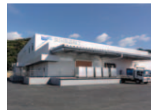
Marine product processing plant of a reconstruction loan recipient
