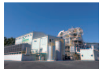
Electric power station of a Fund recipient
