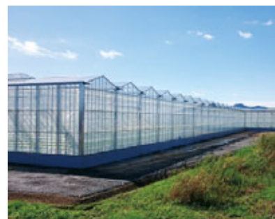
Plant factory of a reconstruction fund recipient
