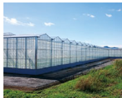
Plant factory of a reconstruction fund recipient
