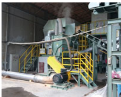
Lumber processing facility of a reconstruction loan recipient
