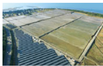
Solar power generation facility of a fund recipient
