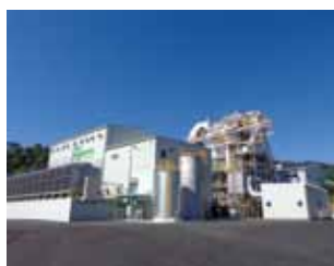
Power station of a fund recipient
